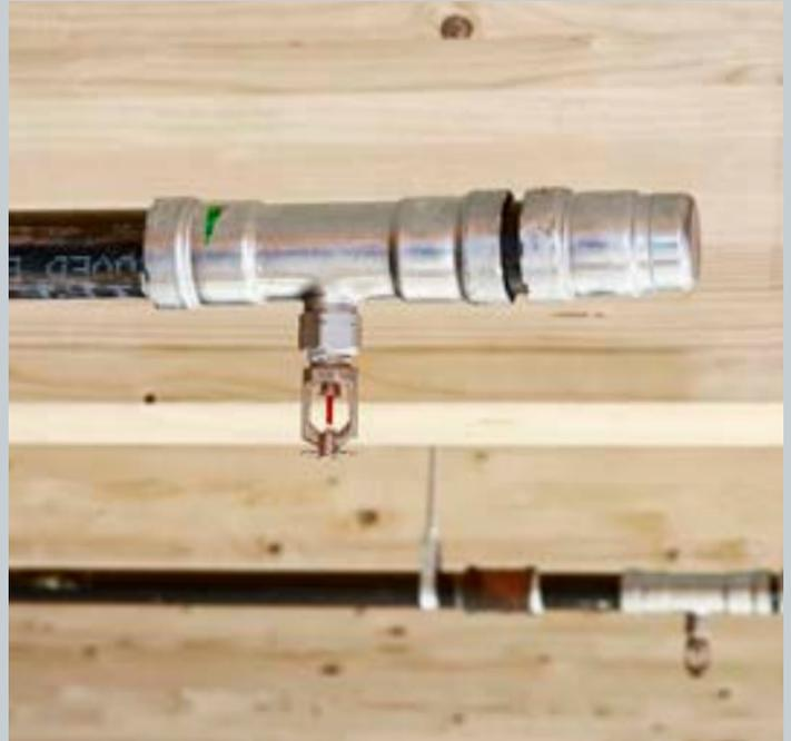
Viega MegaPress is UL and FM certified for fire protection applications in sizes ½" to 2". As with other Viega press systems, Viega MegaPress fittings can be used in pre-fabricated assemblies, producing a straight, clean installation. And with patented Smart Connect technology, installers can verify that all fittings in pre-fabbed assemblies are secure.
